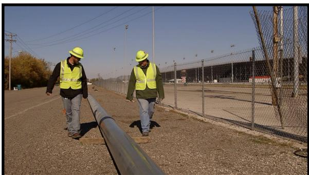
Ameren Illinois enhanced natural gas service by upgrading a high-pressure distribution gas pipe that runs adjacent to Gateway Motorsports Park. The new 12-inch coated steel pipe will fully protect the pipeline from corrosion while allowing for increased system capacity, safety, and reliability to the residential, commercial, and industrial customers served in Madison, East St. Louis and surrounding areas.
