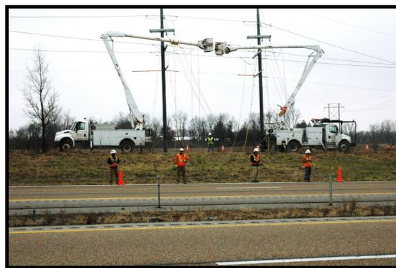
J.F. Electric crew members working on the new Ameren Illinois substation in Collinsville safely pulled power lines across all lanes of Interstates 55-70 to be hooked up to the substation. The substation added capacity to meet increasing customer load growth in the three communities while reinforcing the existing electric system in Madison County and enhance service reliability.
